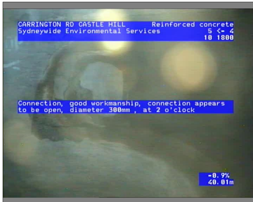
Photo: 093503_18022022_A.JPG, Media No.: LTS LOCKLEY,_0, 00:01:58 40.01m, Connection, good workmanship, connection appears to be open, diameter 300mm , at 2 o'clock
