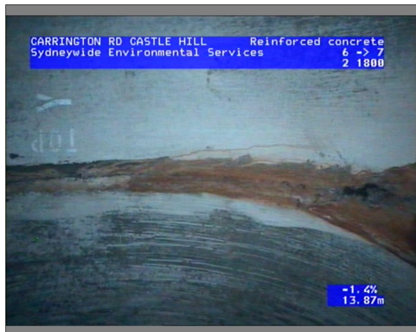
Photo: 075851_18022022_B.JPG, Media No.: LTS LOCKLEY,_0, 00:01:07 13.87m, Infiltration, sweating , from 12 to 12 o'clock
