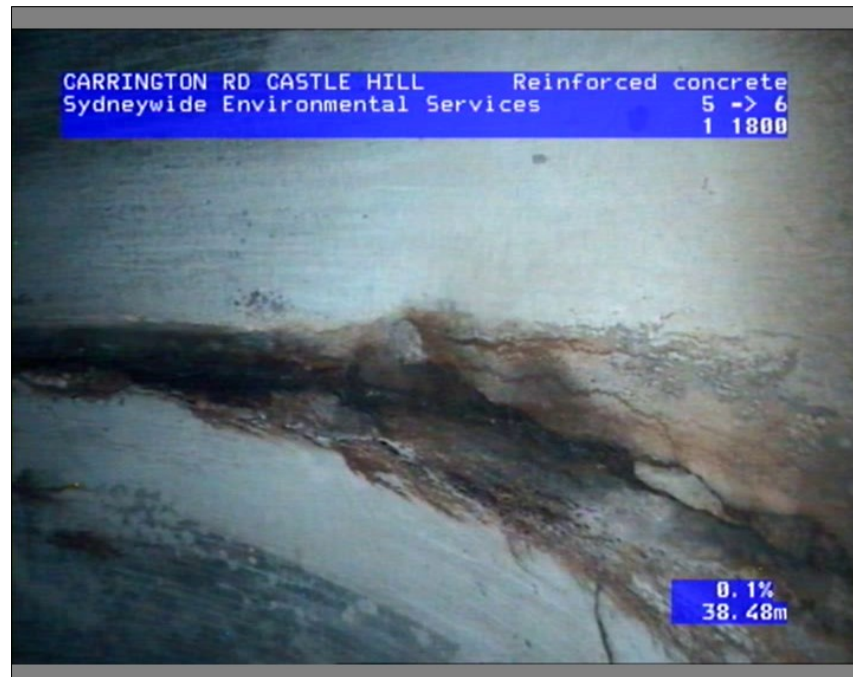
Photo: 075414_18022022_A.JPG, Media No.: LTS LOCKLEY,_0, 00:03:46 38.48m, Infiltration, sweating , from 2 to 5 o'clock
