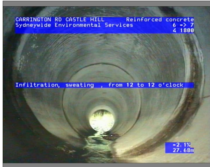
Photo: 082521_18022022_A.JPG, Media No.: LTS LOCKLEY,_0, 00:02:38 27.66m, Infiltration, sweating , from 12 to 12 o'clock
