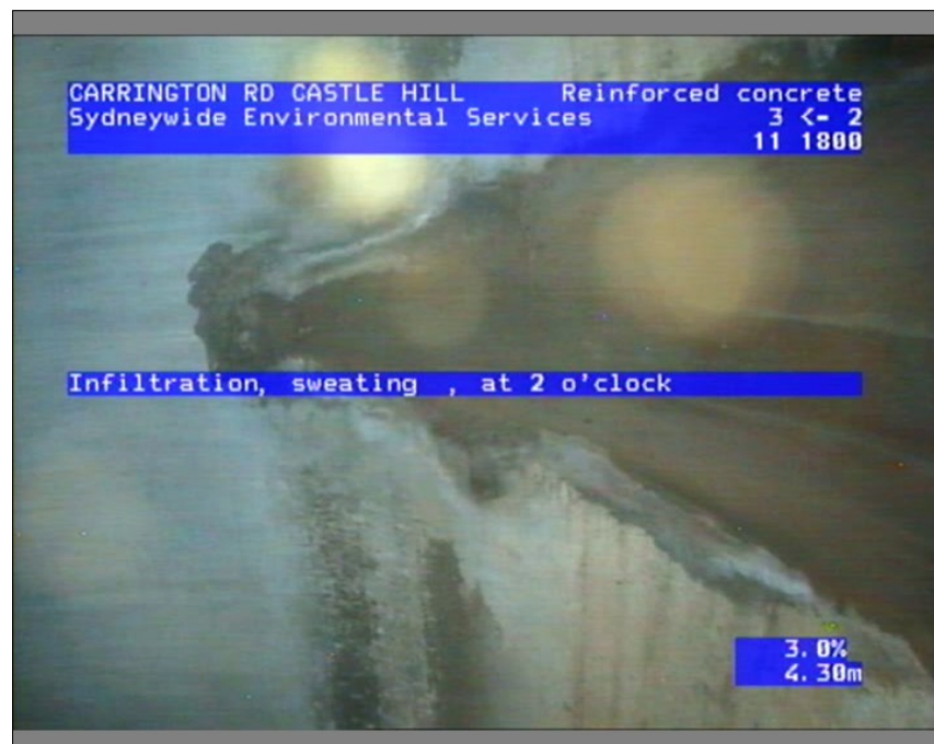
Photo: 094754_18022022_A.JPG, Media No.: LTS LOCKLEY,_0, 00:00:42 4.3m, Infiltration, sweating , at 2 o'clock
