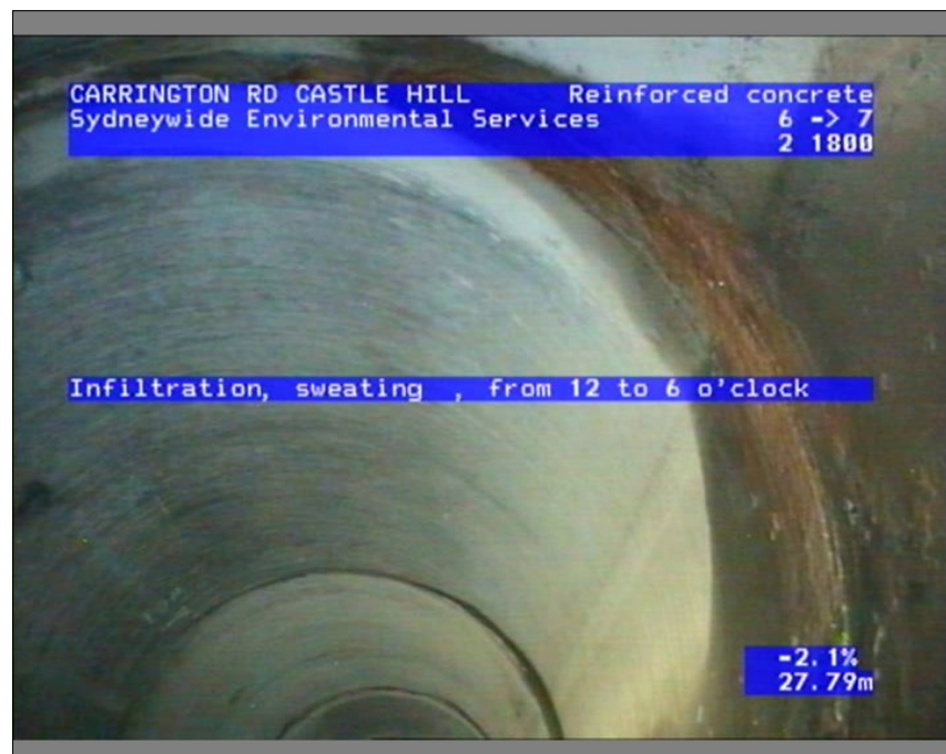
Photo: 080015_18022022_A.JPG, Media No.: LTS LOCKLEY,_0, 00:02:21 27.73m, Infiltration, sweating , from 12 to 6 o'clock
