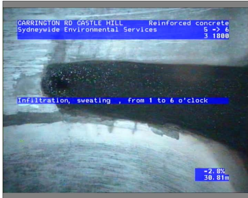
Photo: 081554_18022022_A.JPG, Media No.: LTS LOCKLEY,_0, 00:02:21 31.09m, Infiltration, sweating , from 1 to 6 o'clock
