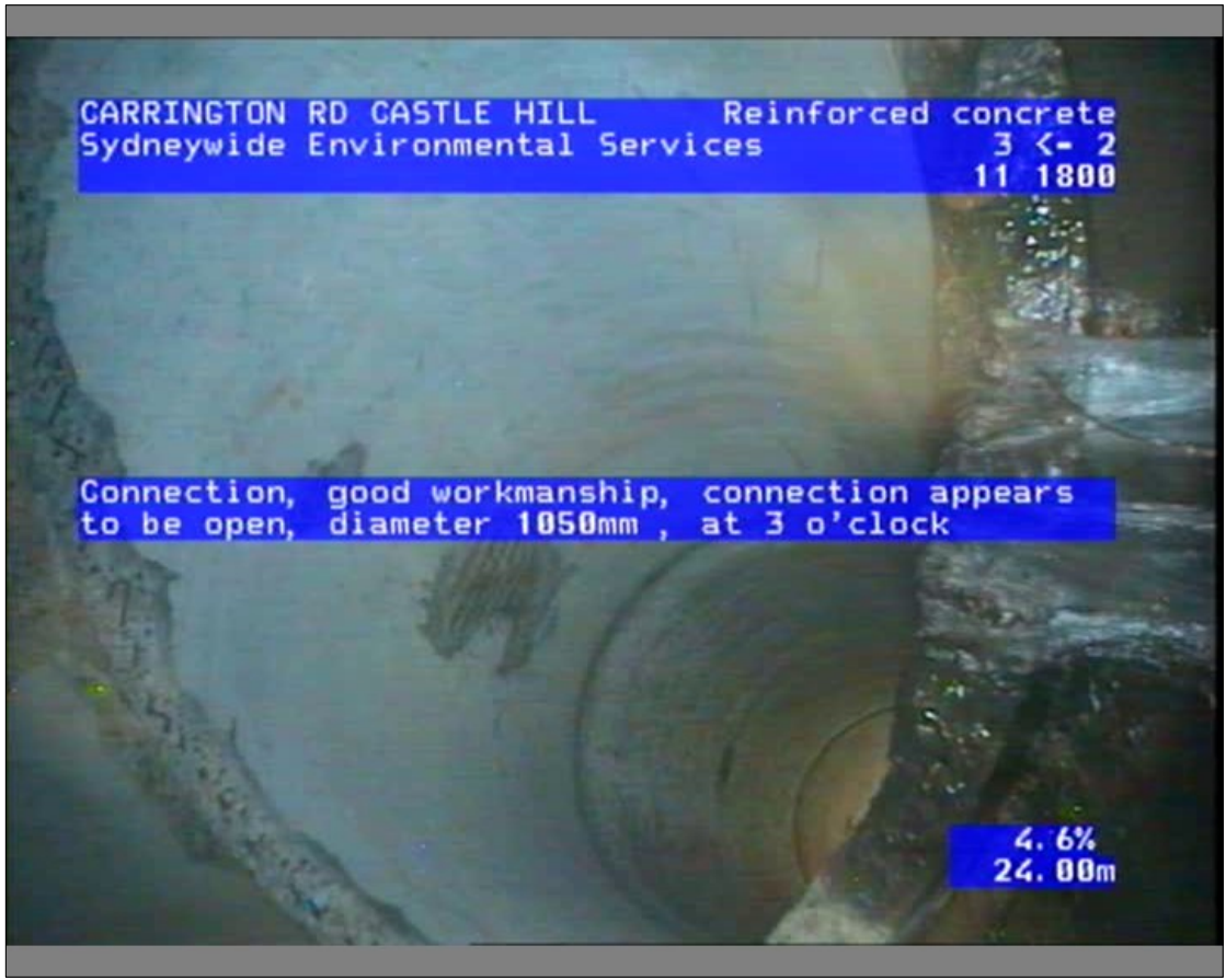
Photo: 095129_18022022_A.JPG, Media No.: LTS LOCKLEY_0, 00:03:11 24m, Connection, good workmanship, connection appears to be open, diameter 1050mm, at 3 o'clock
