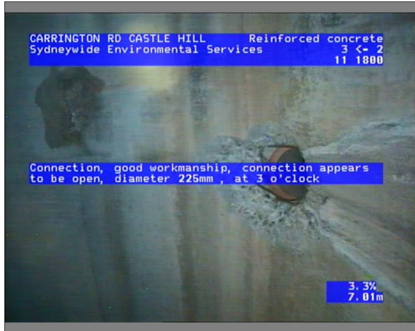
Photo: 094830_18022022_A.JPG, Media No.: LTS LOCKLEY,_0, 00:01:05 7.01m, Connection, good workmanship, connection appears to be open, diameter 225mm , at 3 o'clock
