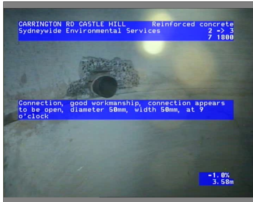
Photo: 085944_18022022_A.JPG, Media No.: LTS LOCKLEY,_0, 00:00:25 3.58m, Connection, good workmanship, connection appears to be open, diameter 50mm, width 50mm, at 9 o'clock
