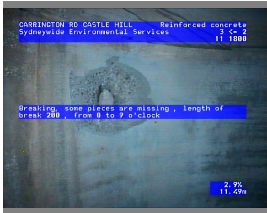
Photo: 094946_18022022_A.JPG, Media No.: LTS LOCKLEY,_0, 00:01:50 11.49m, Breaking, some pieces are missing, length of break 200, from 8 to 9 o'clock
