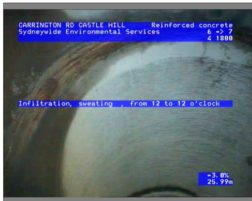
Photo: 082506_18022022_A.JPG, Media No.: LTS LOCKLEY,_0, 00:02:25 25.99m, Infiltration, sweating , from 12 to 12 o'clock
