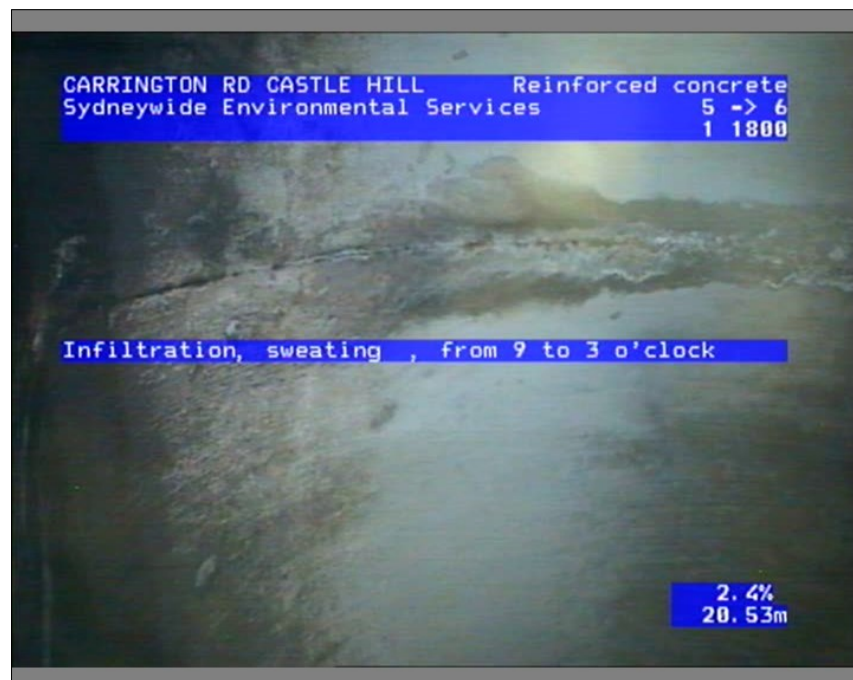
Photo: 075222_18022022_A.JPG, Media No.: LTS LOCKLEY,_0, 00:02:13 20.53m, Infiltration, sweating , from 9 to 3 o'clock
