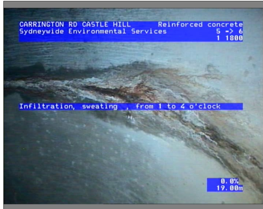
Photo: 075134_18022022_A.JPG, Media No.: LTS LOCKLEY,_0, 00:01:30 19m, Infiltration, sweating , from 1 to 4 o'clock
