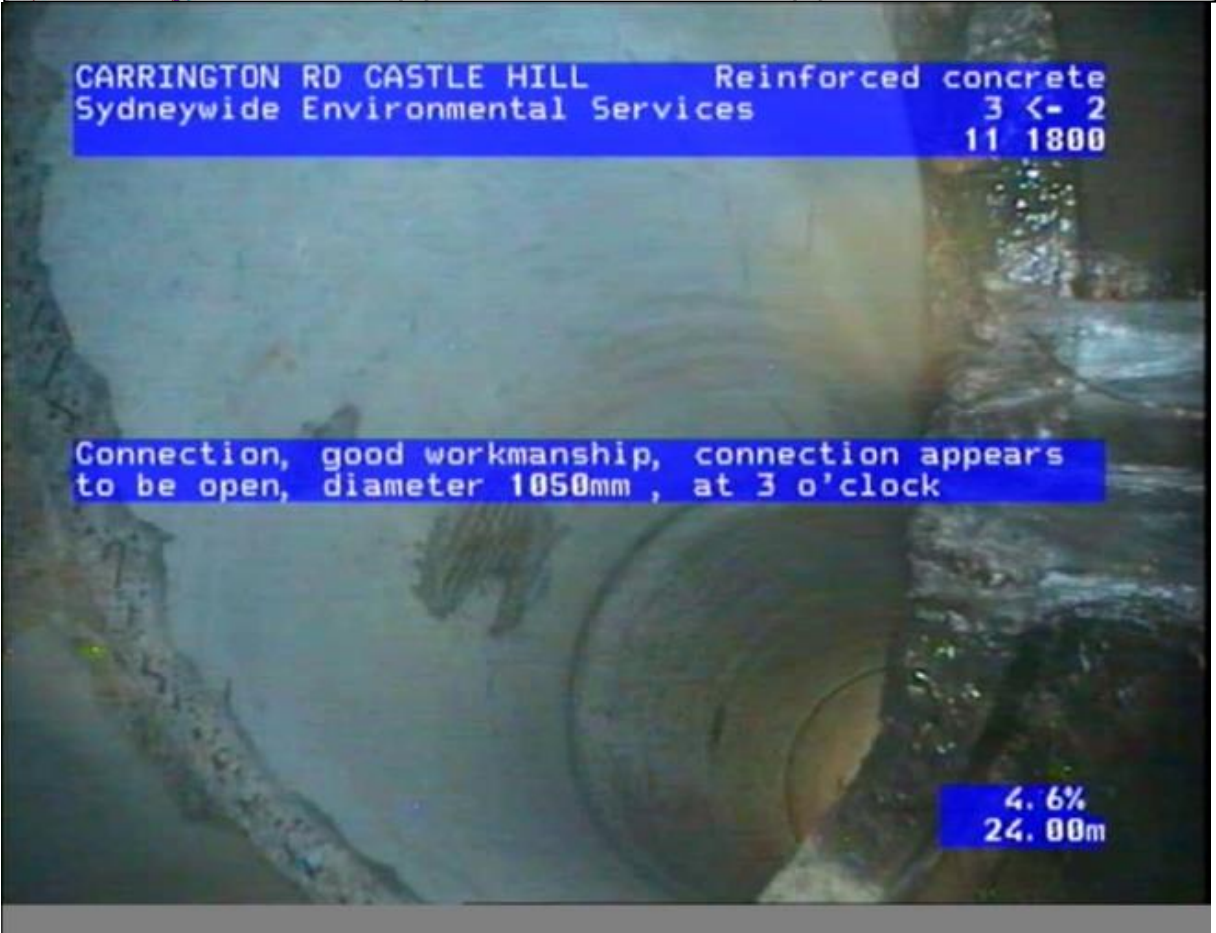
Figure 5. Open connections 1050 mm diameter
