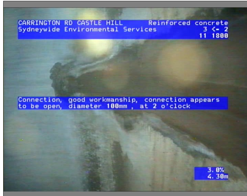
Photo: 094745_18022022_A.JPG, Media No.: LTS LOCKLEY,_0, 00:00:38 4.3m, Connection, good workmanship, connection appears to be open, diameter 100mm , at 2 o'clock
