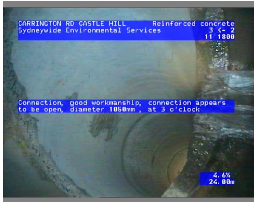
Photo: 095129_18022022_A.JPG, Media No.: LTS LOCKLEY,_0, 00:03:11 24m, Connection, good workmanship, connection appears to be open, diameter 1050mm , at 3 o'clock
