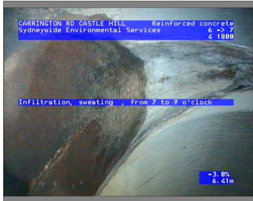
Photo: 081936_18022022_A.JPG, Media No.: LTS LOCKLEY,_0, 00:00:39 6.41m, Infiltration, sweating , from 7 to 9 o'clock
