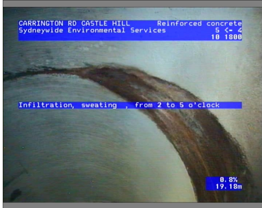
Photo: 093357_18022022_A.JPG, Media No.: LTS LOCKLEY,_0, 00:00:58 19.18m, Infiltration, sweating , from 2 to 5 o'clock
