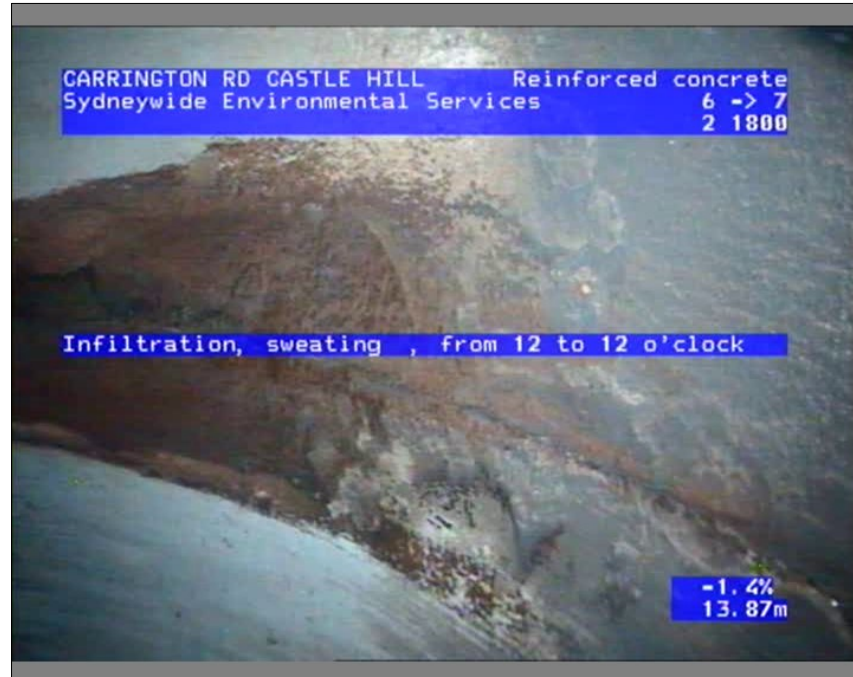
Photo: 075845_18022022_A.JPG, Media No.: LTS LOCKLEY,_0, 00:01:07 13.87m, Infiltration, sweating , from 12 to 12 o'clock
