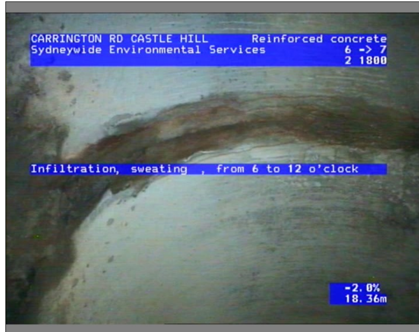
Photo: 075920_18022022_A.JPG, Media No.: LTS LOCKLEY,_0, 00:01:37 18.16m, Infiltration, sweating , from 6 to 12 o'clock
