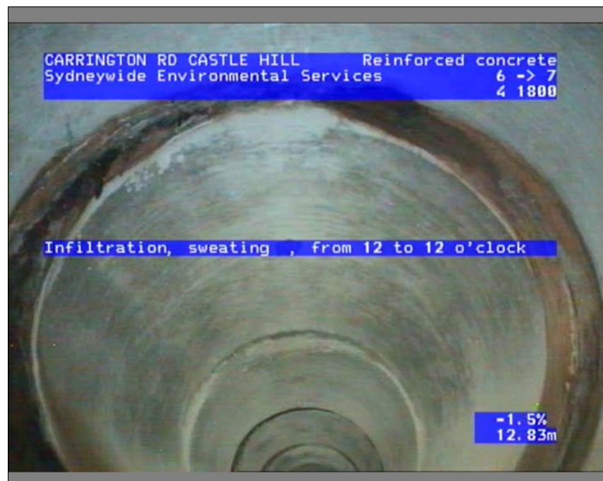
Photo: 082006_18022022_A.JPG, Media No.: LTS LOCKLEY,_0, 00:01:06 12.8m, Infiltration, sweating , from 12 to 12 o'clock
