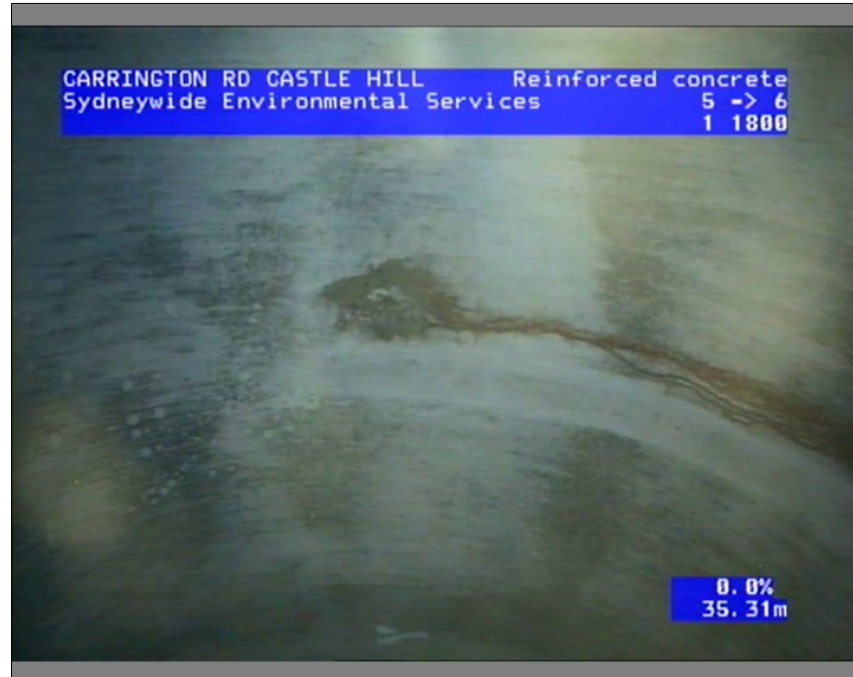
Photo: 075327_18022022_A.JPG, Media No.: LTS LOCKLEY,_0, 00:03:11 35.32m, Infiltration, sweating , at 12 o'clock
