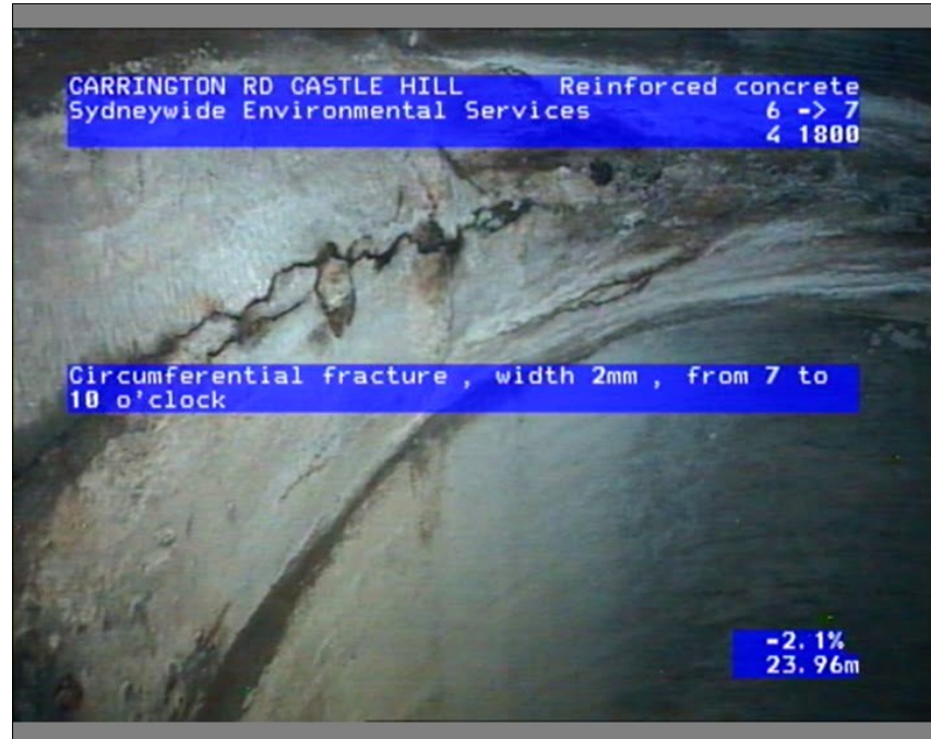
Photo: 082125_18022022_A.JPG, Media No.: LTS LOCKLEY,_0, 00:02:03 23.96m, Circumferential fracture , width 2mm , from 7 to 10 o'clock
