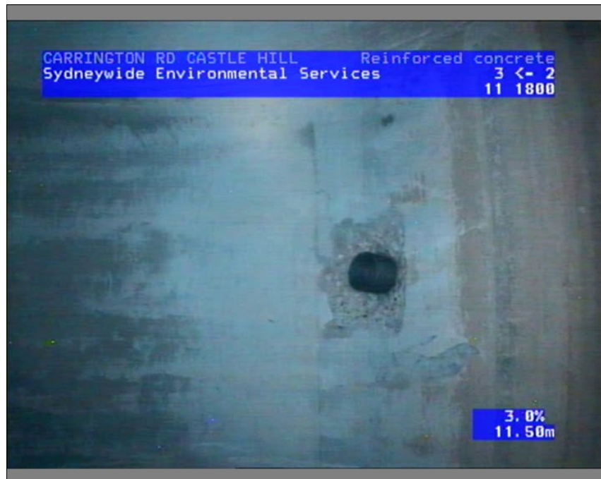
Photo: 095021_18022022_A.JPG, Media No.: LTS LOCKLEY,_0, 00:02:07 11.5m, Connection, good workmanship, connection appears to be open, diameter 50mm, at 3 o'clock
