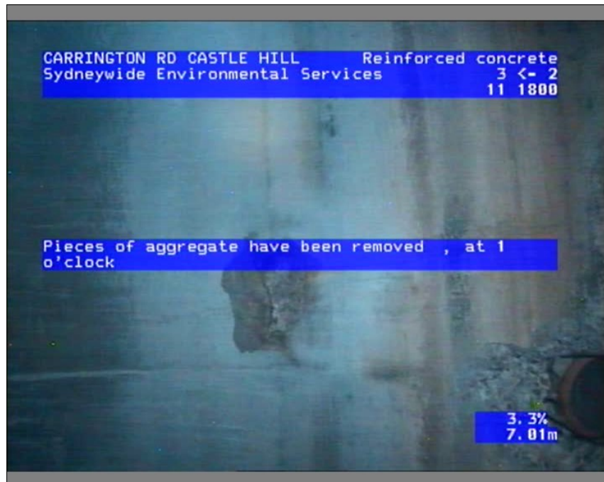
Photo: 094859_18022022_A.JPG, Media No.: LTS LOCKLEY,_0, 00:01:15 7.01m, Pieces of aggregate have been removed , at 1 o'clock
